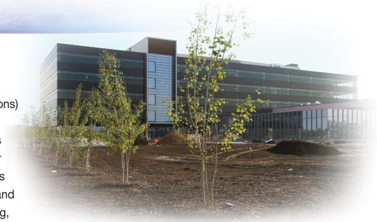
Panduit World Headquarters under construction
